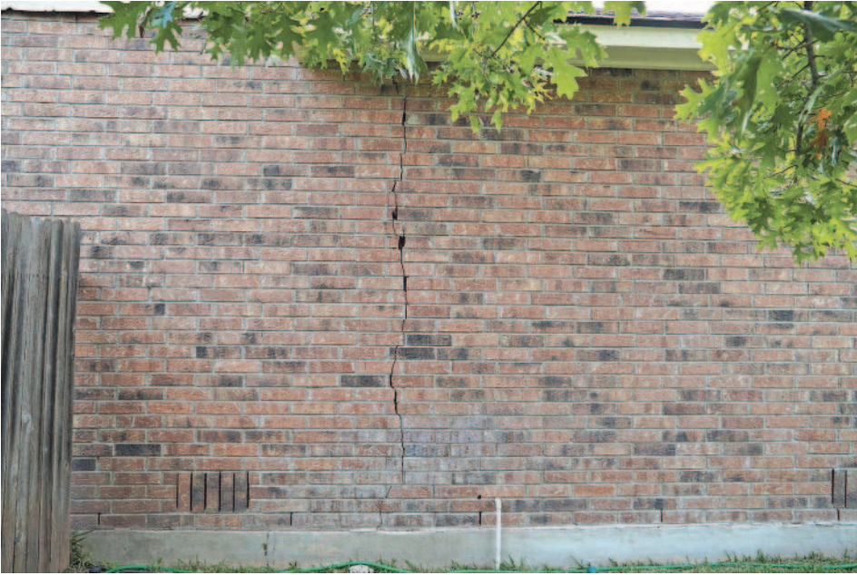
During a drought, soils contract and the ground shrinks, leaving gaps underneath homes. Cracks and other visual signs of foundational instability can appear when the home shifts to fill the gaps, creating unevenness and an unlevel foundation. PROVIDED BY FOUNDATION SUPPORT SPECIALISTS
